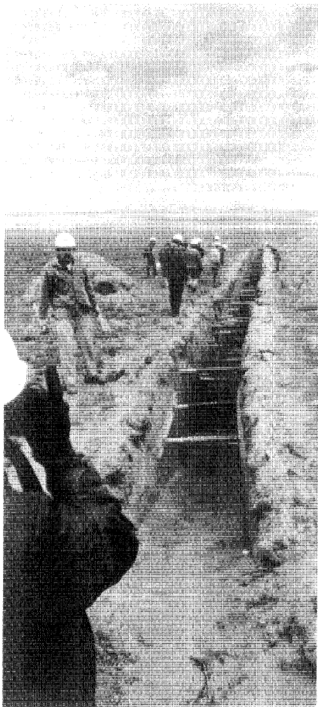
This trench was excavated on the northeast flank of Rattlesnake Mountain at the Hanford (Wash.) reservation to ascertain whether a line of scarps (steep slopes) reportedly seen from an airplane could have been a faultline. The project indicated that it was not.
